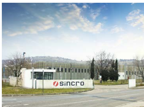
Sincro d.o.o. factory in Škrlevo (Rijeka, CROATIA). Since 2002. Manufacturing of 4 pole industrial alternators (frame sizes from 225 to 500).
