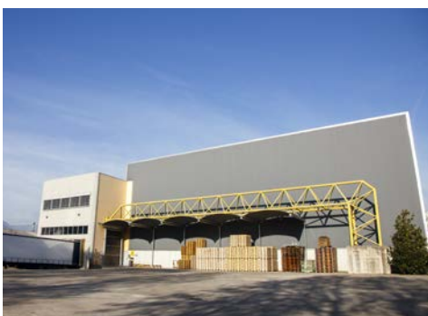
Sincro plant in Cereda di Cornedo (Vicenza, ITALY). Since 1987. Manufacturing of 2 and 4 pole alternators and welders (up to frame size 225).
